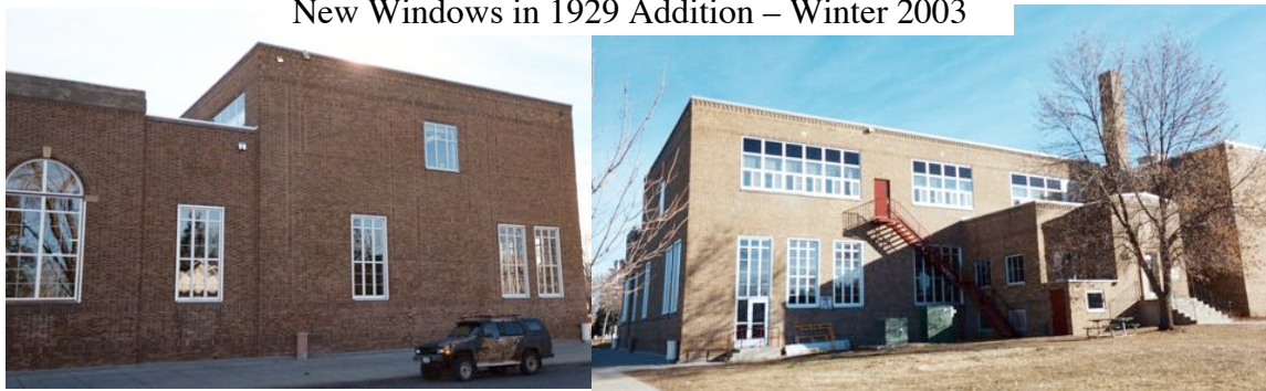
New Windows in 1929 Addition – Winter 2003
